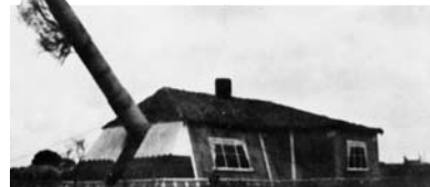
The biggest guns on the whole Atlantic Wall were those of Battery Mirus at Le Frie Baton, Guernsey. The four 30.5cm guns originally came from a First World War Russian battleship. The battery had a range of 32 miles (50km) and controlled the whole of the gulf of St. Malo. This photograph shows a Mirus gun camouflaged as a bungalow.
